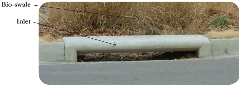
Figure 36: Open Swale Inlet, Topeka, KS
